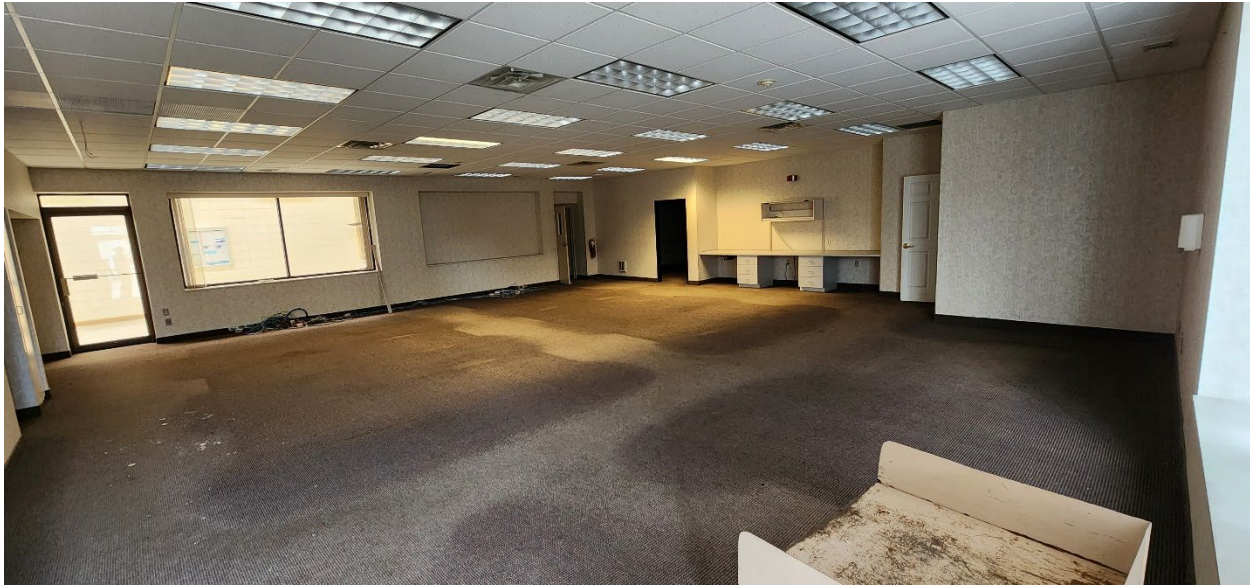
First Floor - Southwest Interior (Original Structure)
