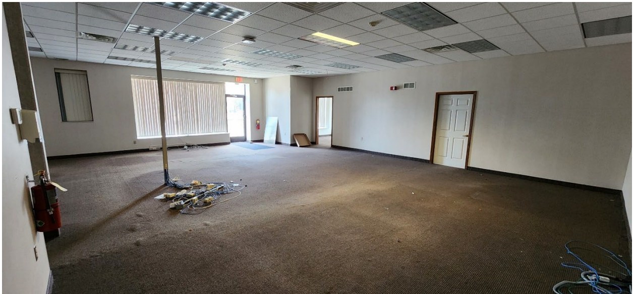
First Floor - Front/West (Original Structure)
