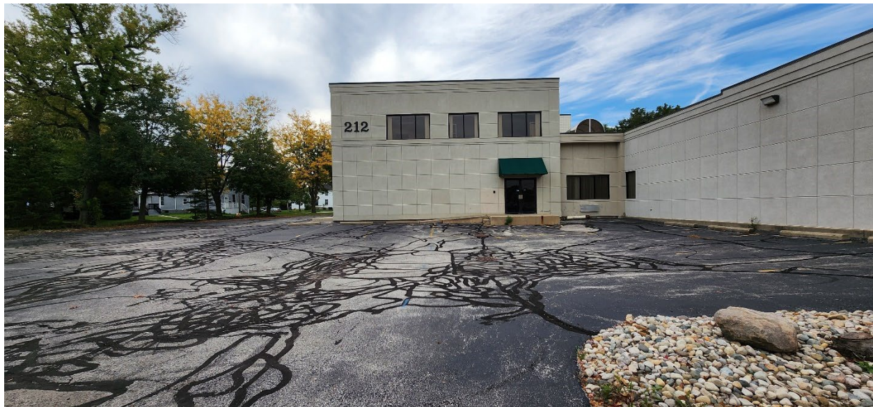
Front View #2 - East
